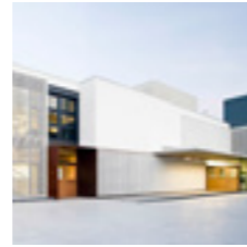
2007 Nuevo Centro St. Peter's School, Barcelona
